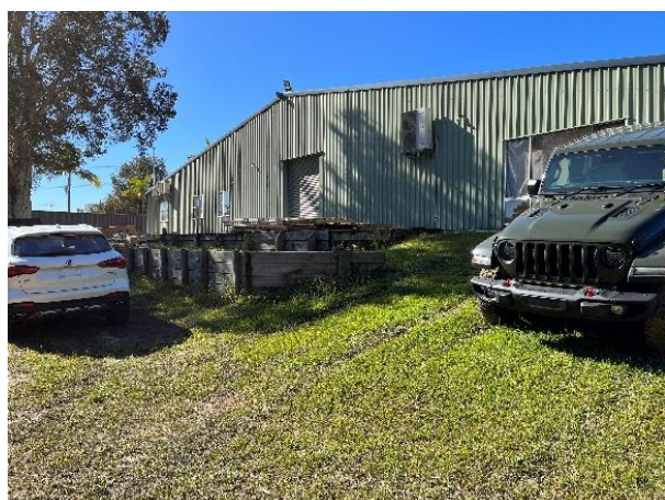
Lot 2: Large metal clad building on raised fill platform.
