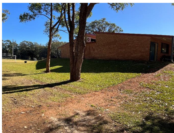
Lot 4: Single storey brick classrooms in east of Lot 4, constructed on 2m high fill embankment. Red clay soils exposed in embankment.
