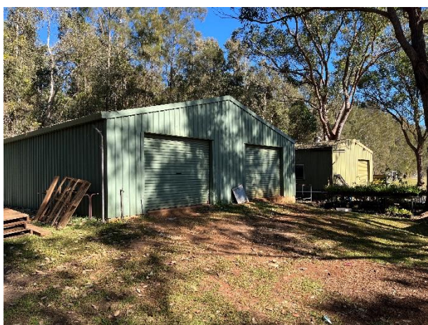
Lot 4 (TP3): Metal sheds located on the southern boundary that appear to be used for storage of maintenance equipment. The sheds are constructed on a 0.5m high fill embankment.
